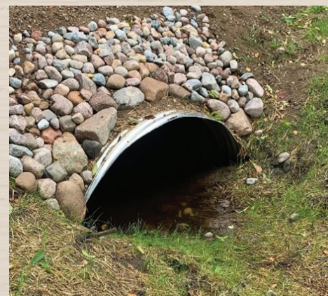
Before (above) and after (below) downstream photos of the newly-installed wetland drainage culvert on Newman Trail Road
